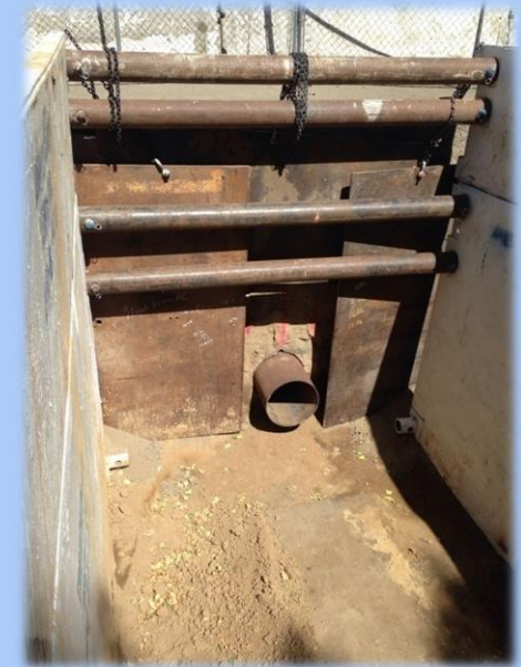
Siphon Replacement Under Highway 395
